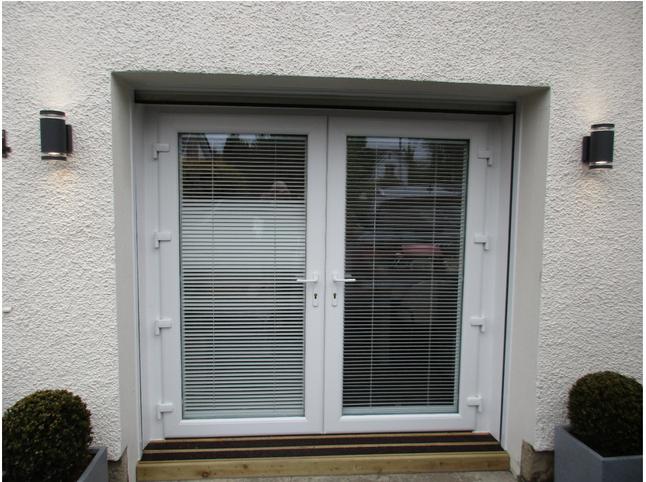
GARAGE FRONTAGE WITH ROLLER SHUTTER RAISED
