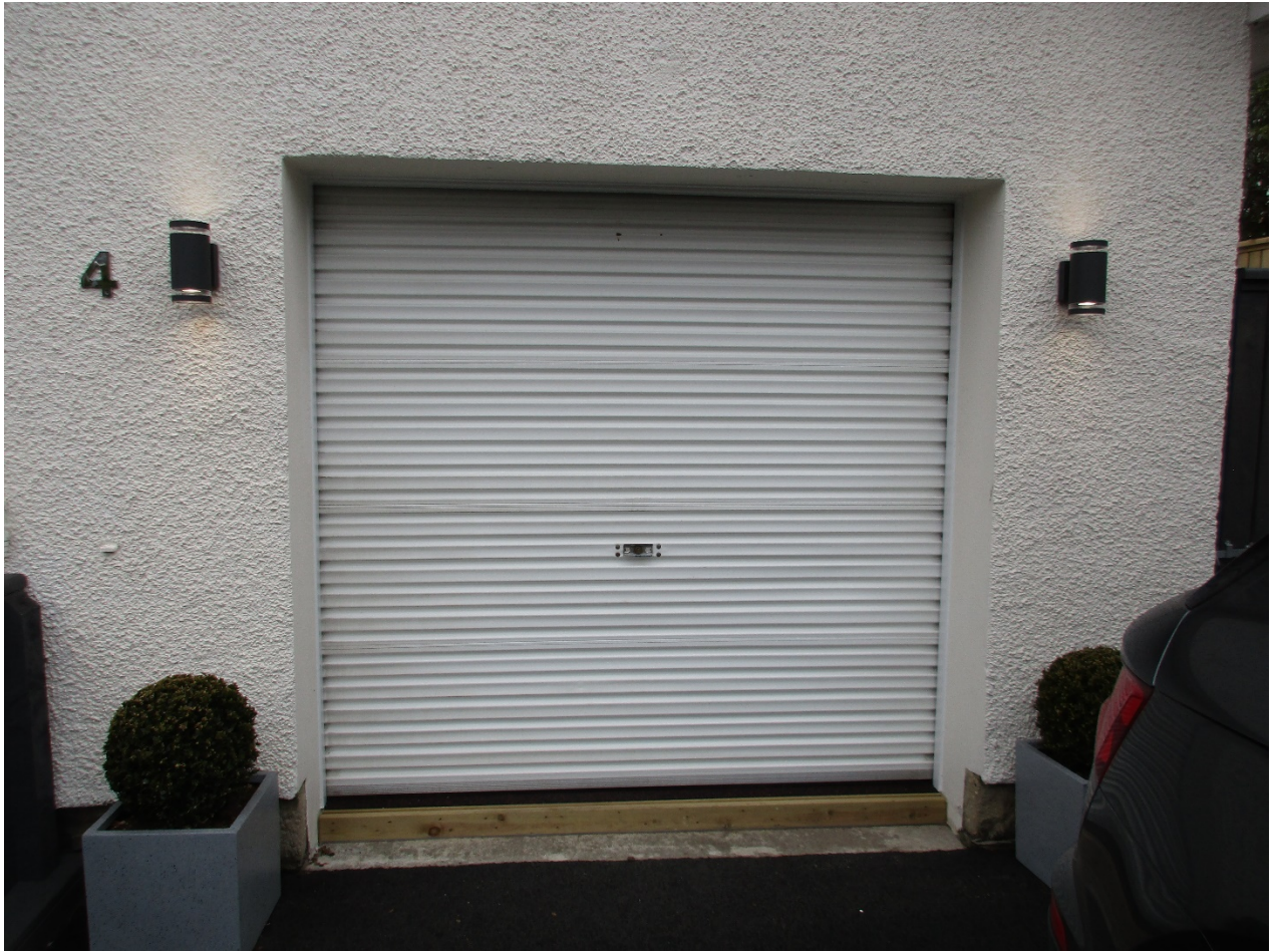
GARAGE FRONTAGE SHOWING ROLLER SHUTTERS CLOSED
